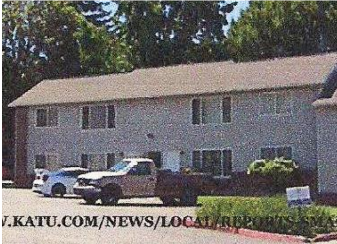
A 3-year old girl fell from this apartment complex
